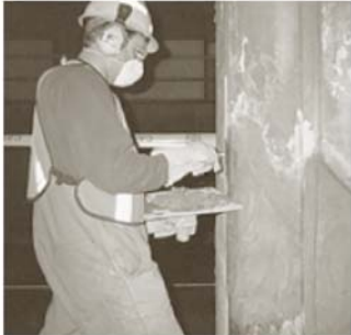
Cementitious General Purpose Repair
