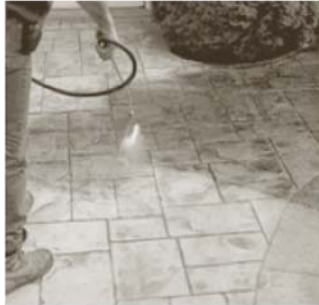
VOC Compliant Curing and Sealing
