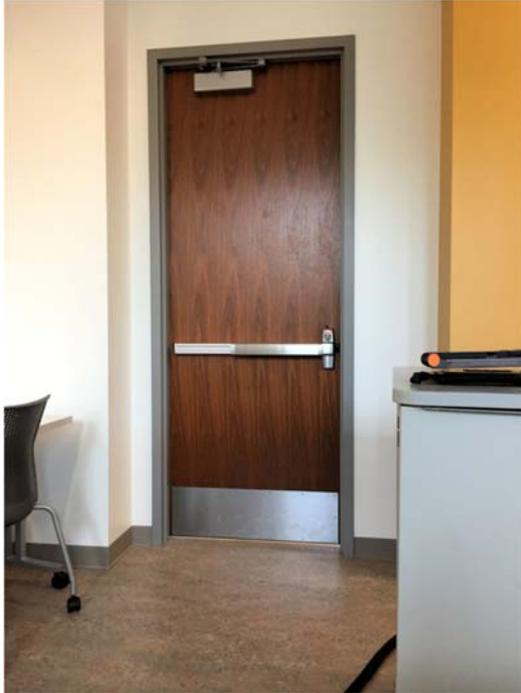
This classroom door on one of our college tours has Von Duprin 99 series panic hardware with the -2 function which allows the outside lever to be locked from the inside. This hardware also has the locked/unlocked indicator (-2SI).
