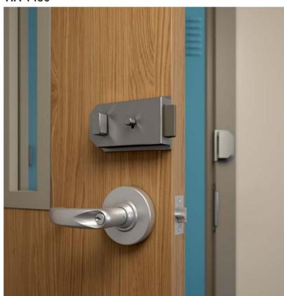
TIA 1436 allows two operations to unlatch an existing classroom door, but the operations can not be simultaneous. The two latching devices shown in this photo are not compliant.
