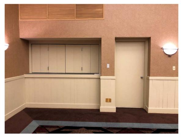
The bottom line is...if a door looks like an egress door it will probably be used as an egress door, and it must comply with the adopted codes. And if a door is not code-compliant, it had better not be a door that is required for egress, or a door that looks like it could be used for egress.
