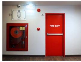
This fire exit door has fire exit hardware, but not all fire exit doors are required to have fire exit hardware. Yes, I'm sure.
