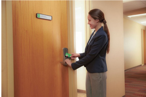
A revision to the 2024 I-Codes clarifies that a door with access control hardware is not considered a special locking arrangement if it is readily openable from the egress side without a key or special
