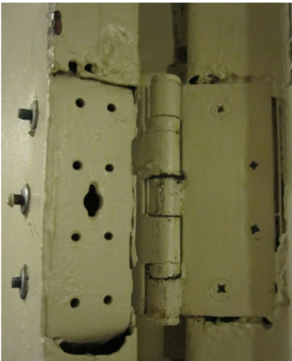
When hinge reinforcements become damaged, creative modifications like this one can result in a non-code-compliant fire door assembly.
