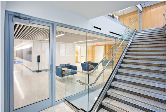
This full-lite fire-resistance-rated glass door offers narrow profile frames to maximize the glazing area along the project's central stairwell. Credit: Courtesy of TGP
