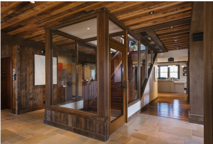
Versatile cover caps allow a wide range of code-compliant design options for fire doors and adjacent assemblies. Credit: Courtesy of TGP
