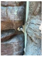
This area was constructed to look like stone, including the panel on the door. I would have painted the door a coordinating color, but with regard to codes, it's ok to disguise the door this way because the "stone" was on the access side of the door leading to an employee area. This wouldn't be allowed if it was the egress side of a door in the path of egress.
