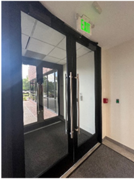
This entry door on an office building has electromagnetic locks mounted at the top of the door, a sensor near the exit sign, and an auxiliary push button on the wall.
