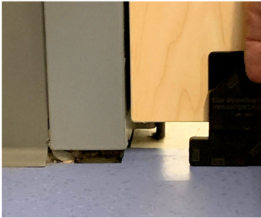
When measuring the clearances on fire door assemblies, it's important to use a gauge or tool that can accurately measure the gaps. Photo: Hal Kelton
