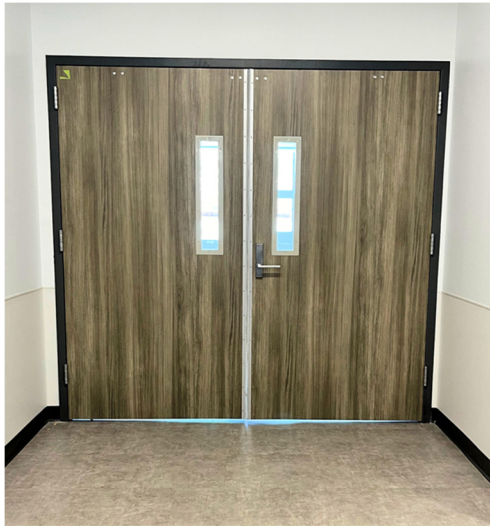
The clearance under this existing pair of fire doors varies from the jambs to the meeting stiles. Photo: Hal Kelton
