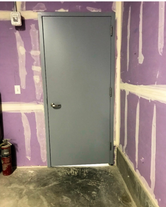
The clearance under this fire door looks like it is in excess of 3/4 inch at the hinge jamb. Photo: Hal Kelton
